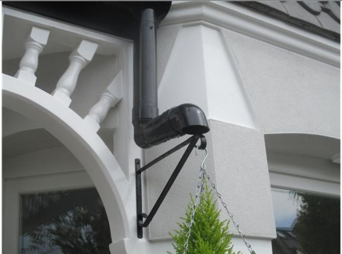
FRONT DOWNPIPE DISCHARGING INTO THIN AIR
