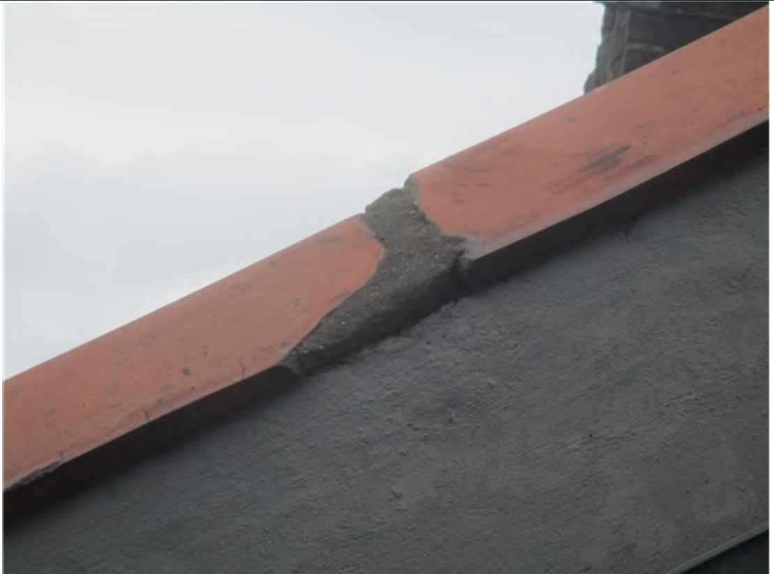
REPAIRED RIDGE TILE CAPPING ON TOP OF PARAPET WALL
