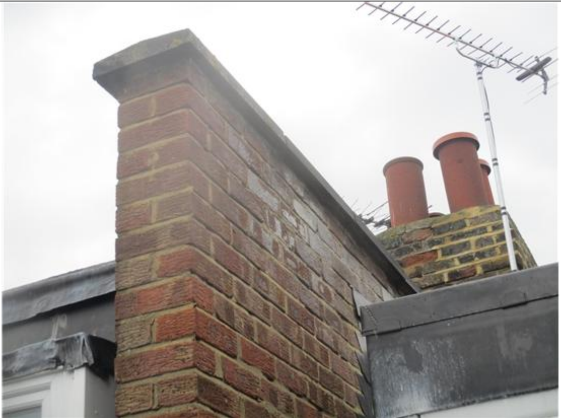
CONCRETE CAPPINGS TO REAR RIGHT PARAPET WALL OF INADEQUATE WIDTH
