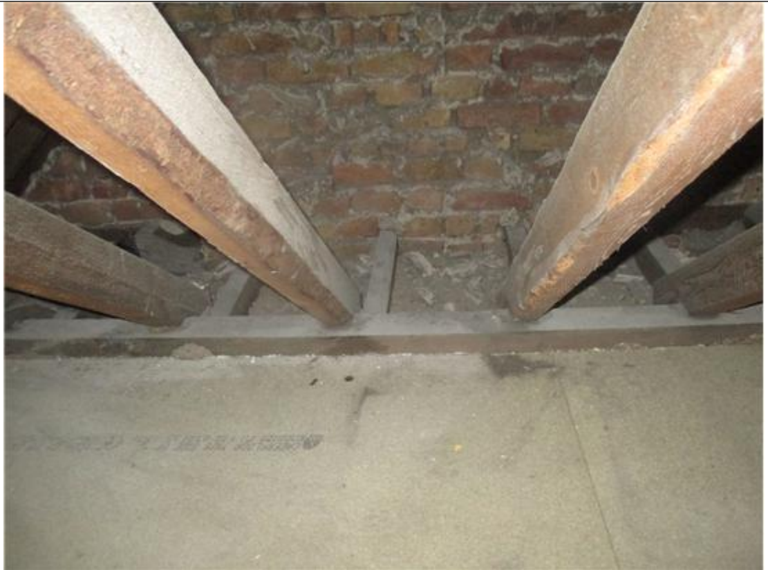
NO INSULATION BETWEEN JOISTS TO FRONT OF ROOF SPACE
