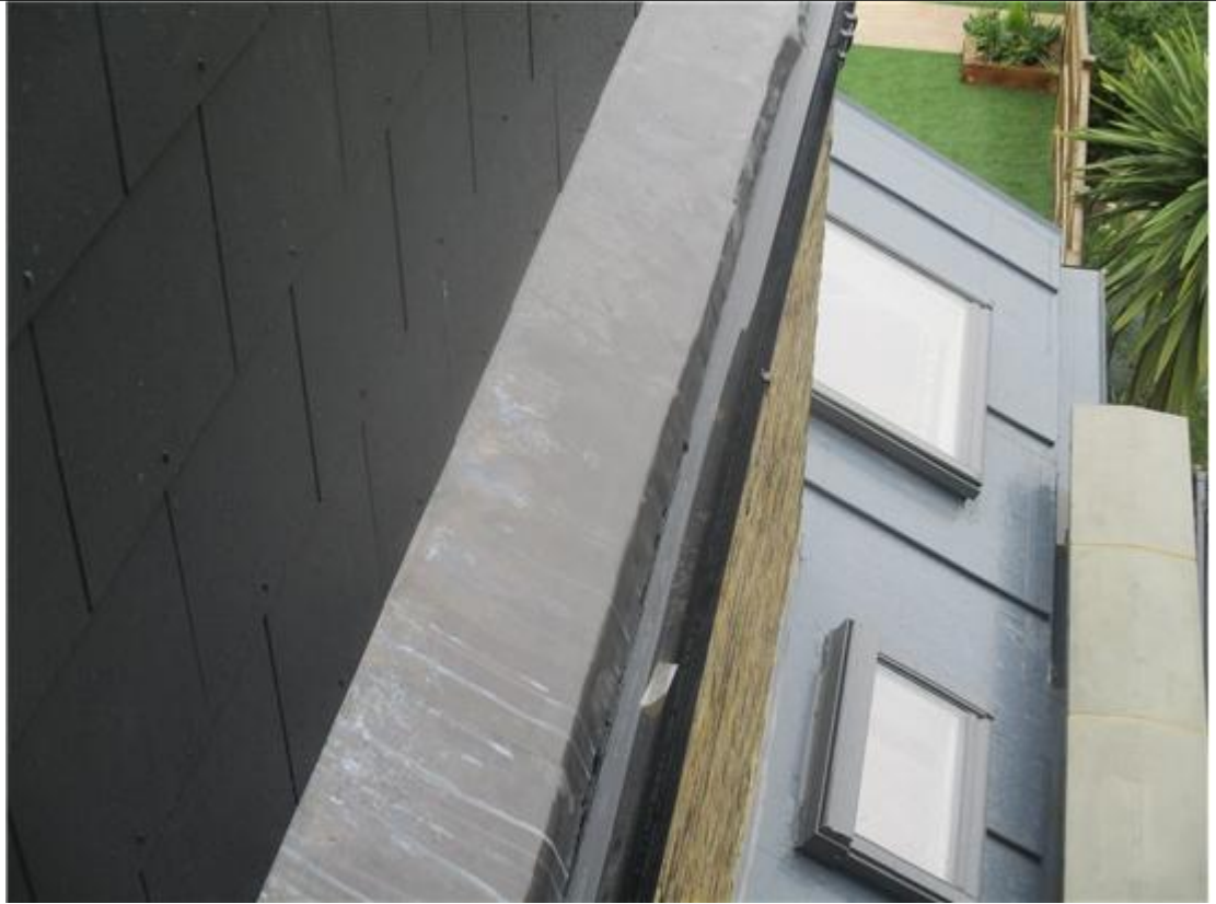
GOOD QUALITY LEADWORK COVERING FOOT OF DORMER
