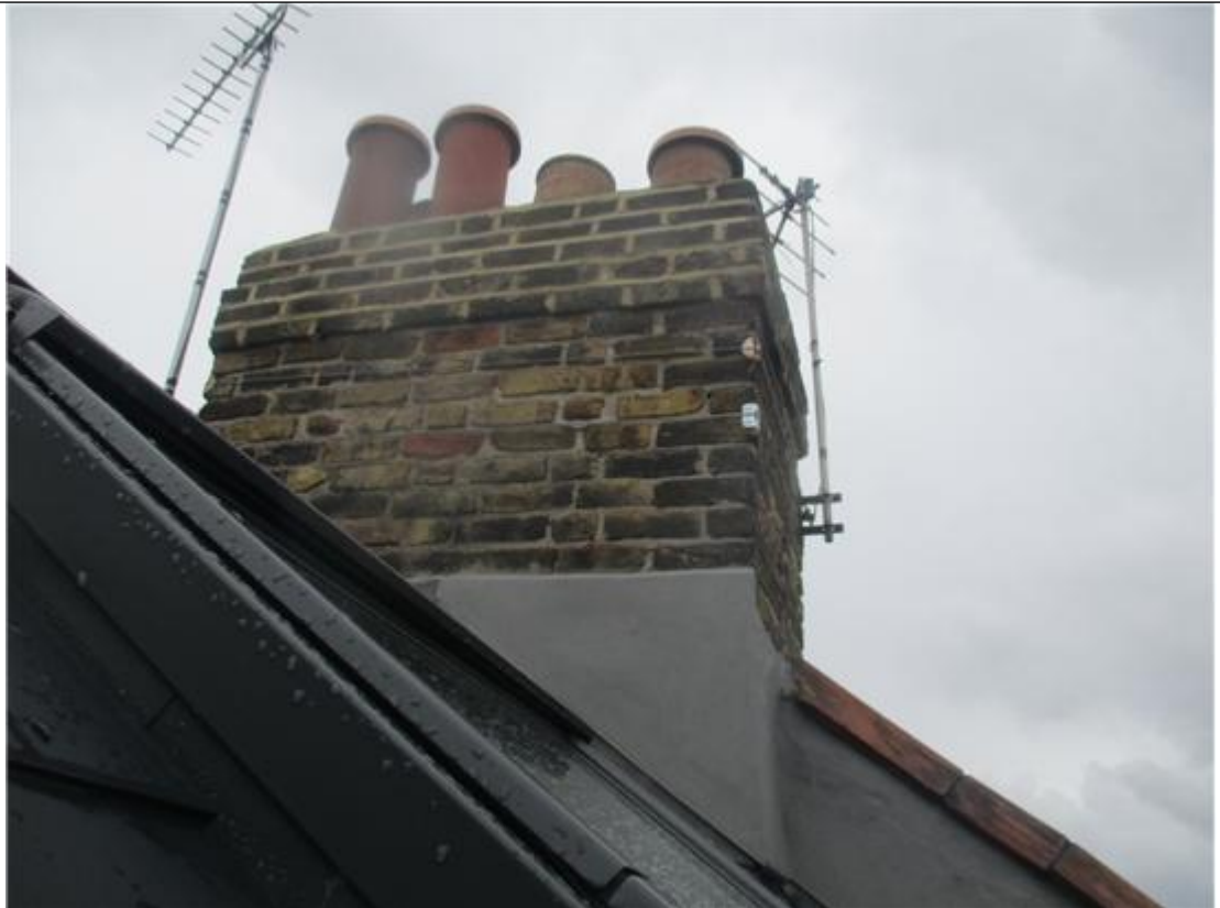
CHIMNEY STACK WITH NO SIGNIFICANT DEFECTS
