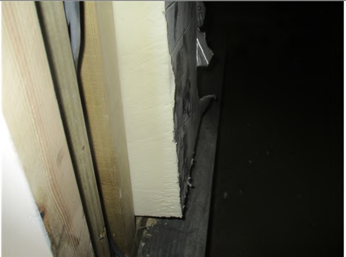
VERTICAL INSULATION BATTS OUT OF POSITION TO ROOF SPACE
