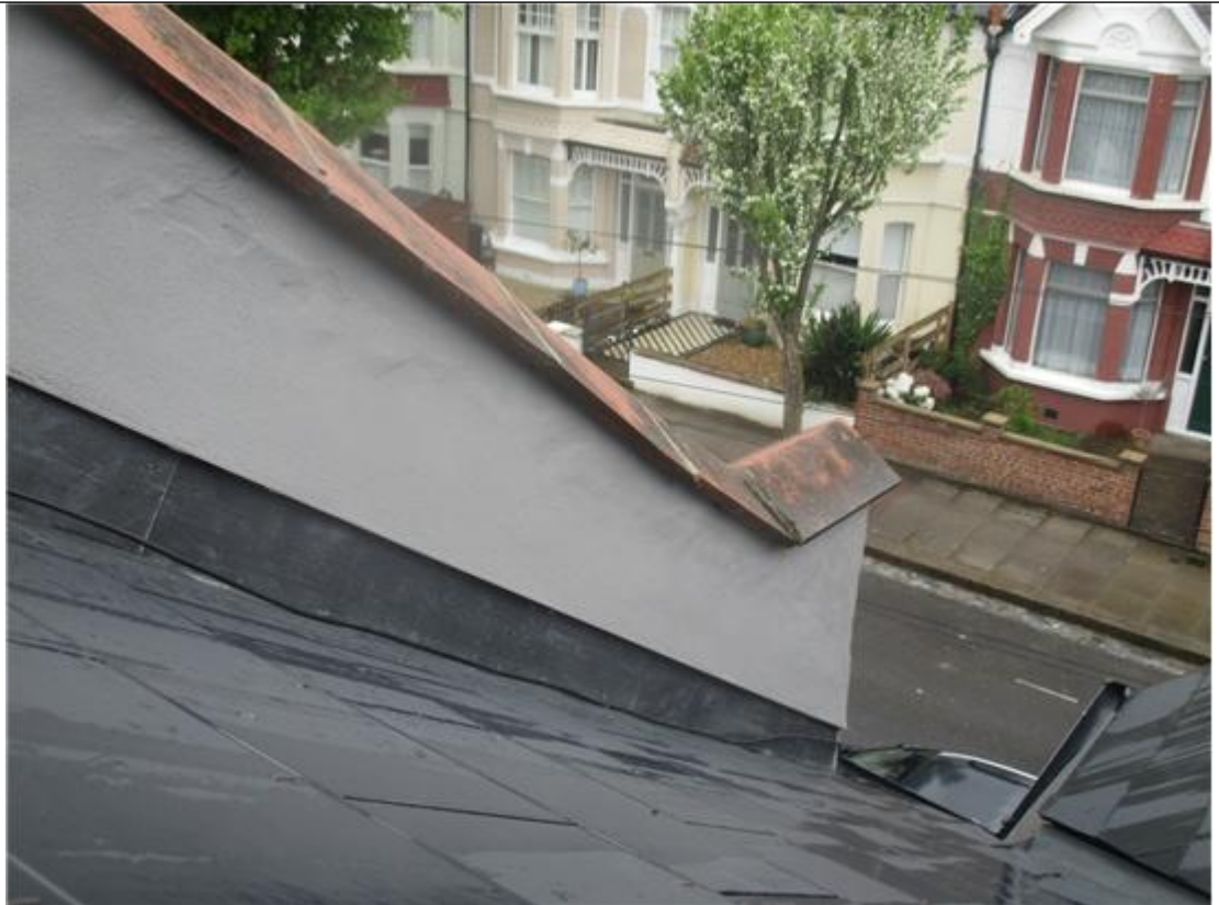
INFERIOR CLAY RIDGE TILES AS THE CAPPING ON THE MAIN ROOF PARAPET WALLS
