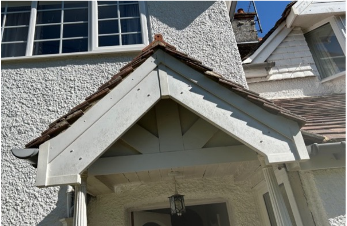
Perimeter PVC boarding to the roof immediately above the front entrance door in satisfactory condition.
