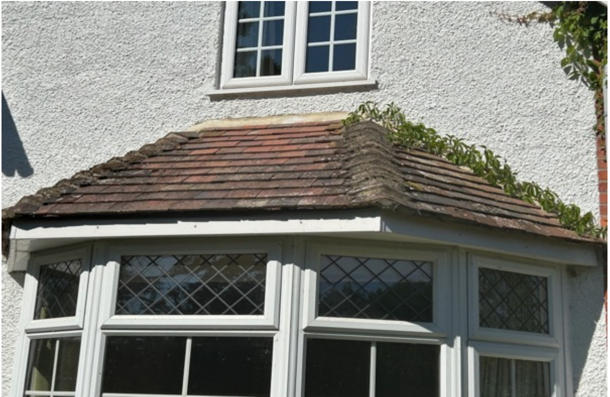
General view of the lower subsidiary bay roof, with no significant defects observed to the tiling.
