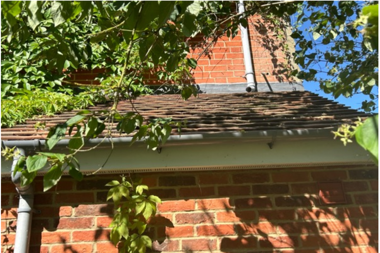
No significant defects noted to the tiling to the rear right subsidiary roof.
