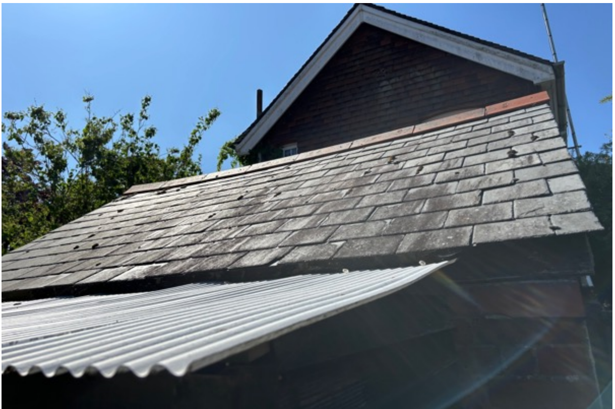
Rear slated slope to the rear outbuilding in fair condition.
