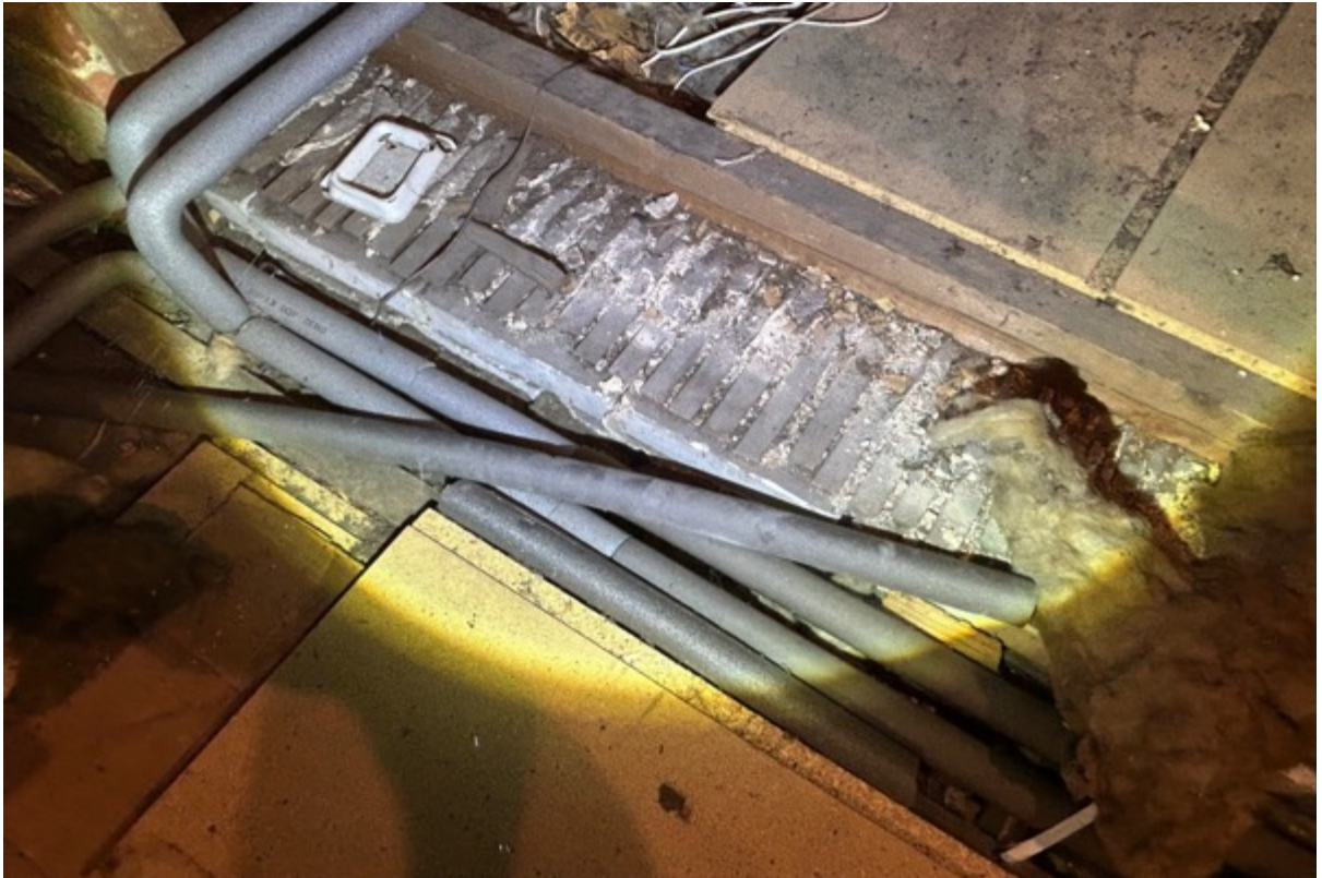
Confirmation that lath and plaster is still present throughout the property as the ceiling finish.
