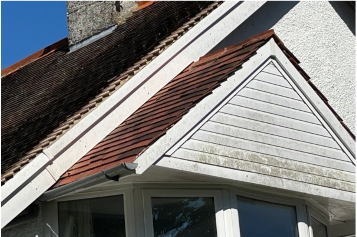
Front slope to the right side upper subsidiary roof in satisfactory condition.
