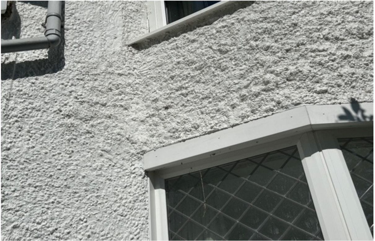
No significant separation between the left side of the taller bay to the right side of the property and the right flank elevation.
