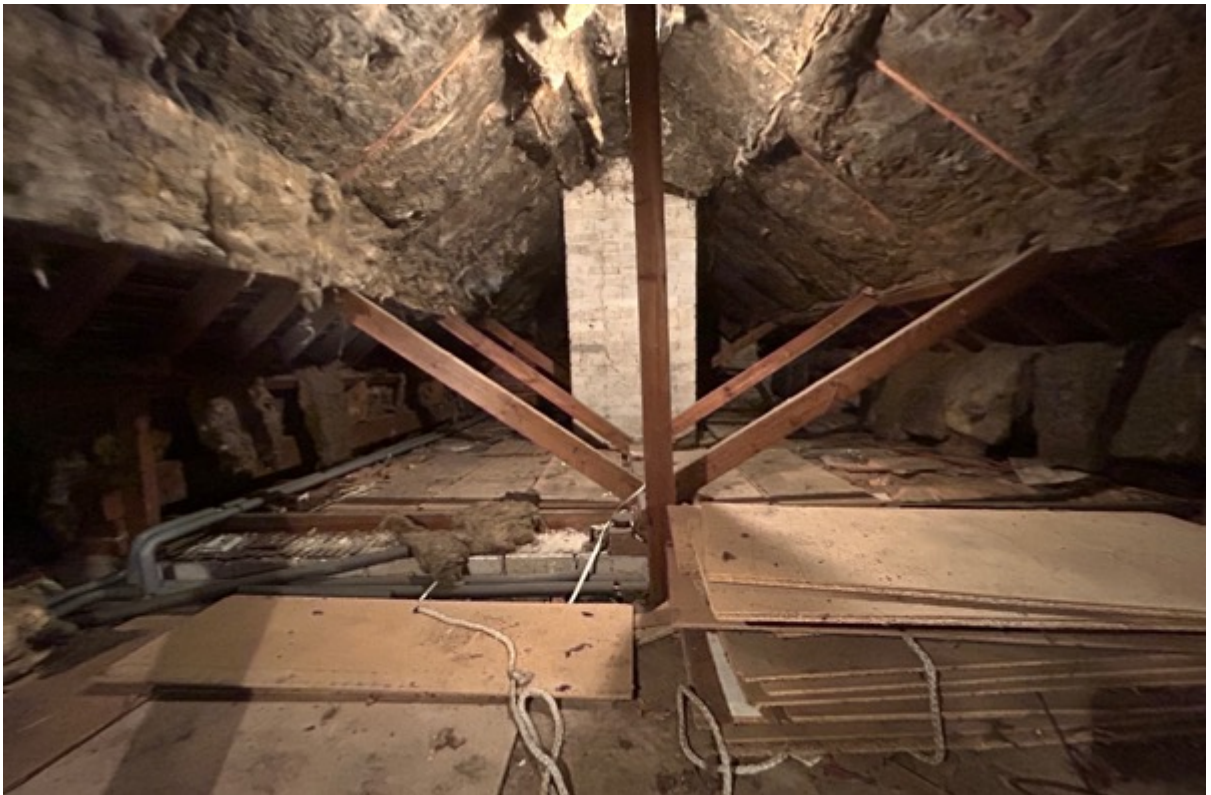
General view of the side-to-side section of the roof space.
