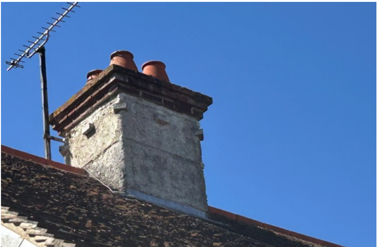
Rear view of the stack.
