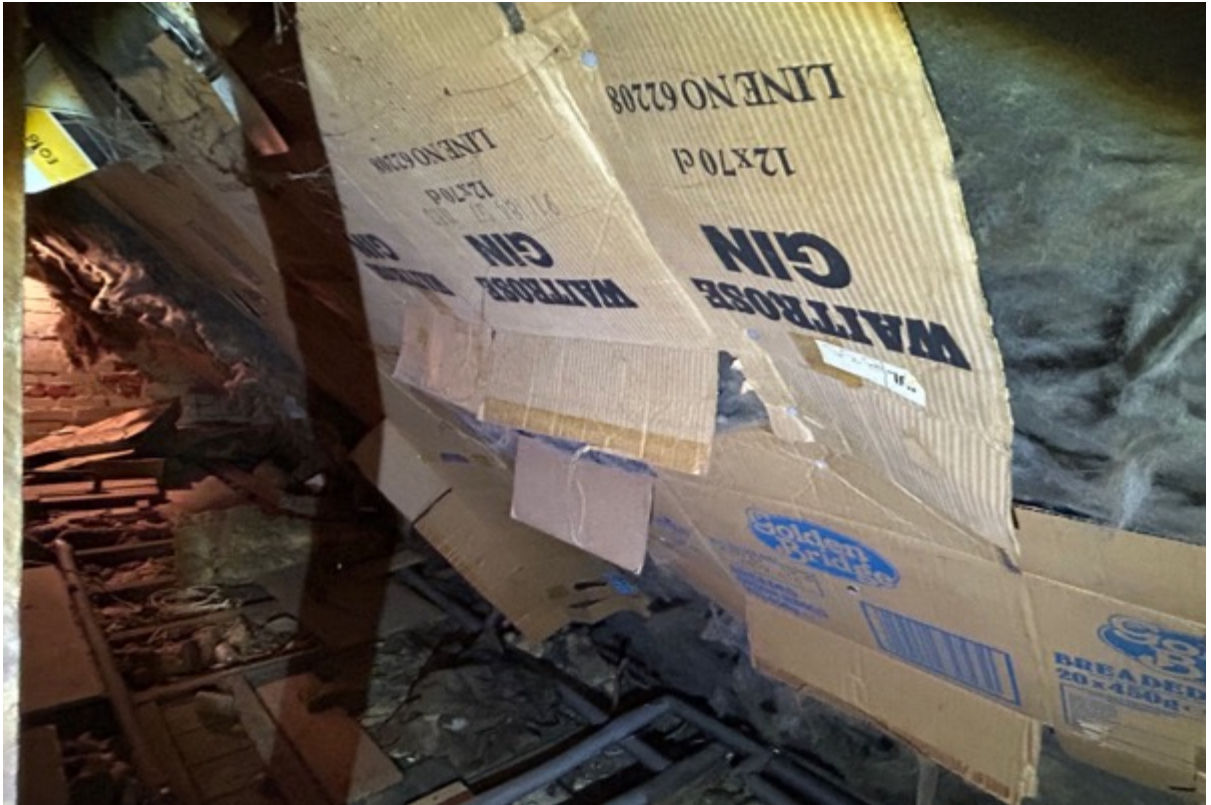
Underside of the rafters covered with cardboard boxes.
