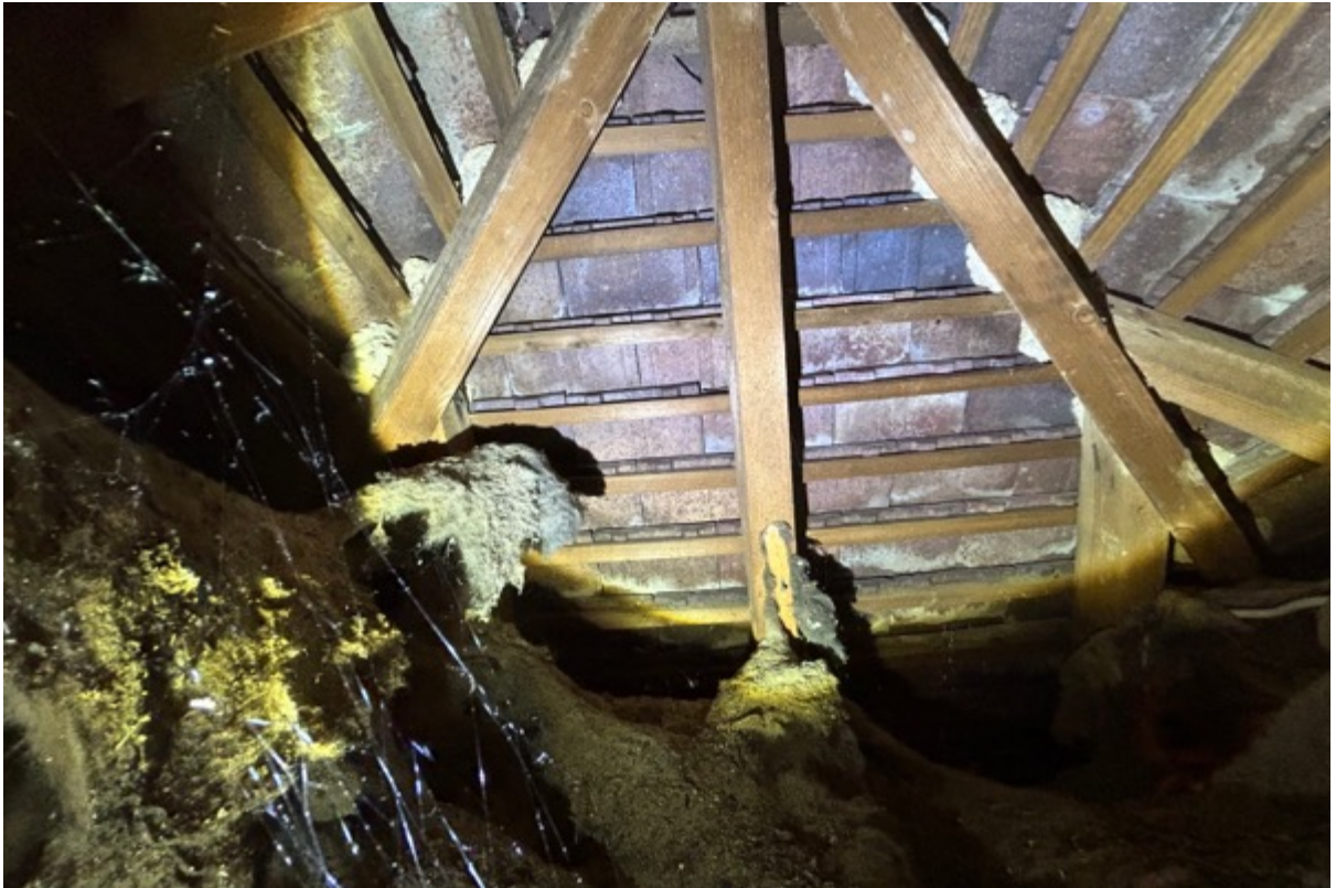
General view of the underside of the roof tiling to the same area.
