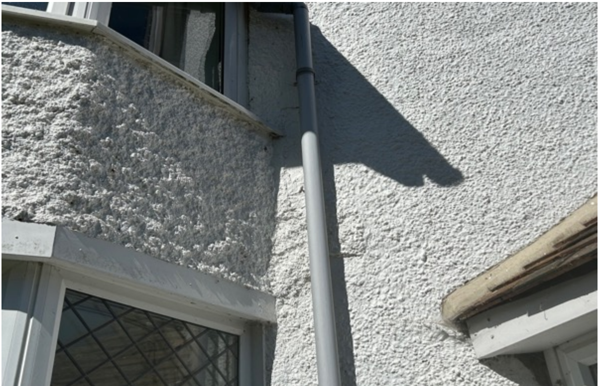
No significant separation between the right side of the taller bay to the right side of the property and the right flank elevation.
