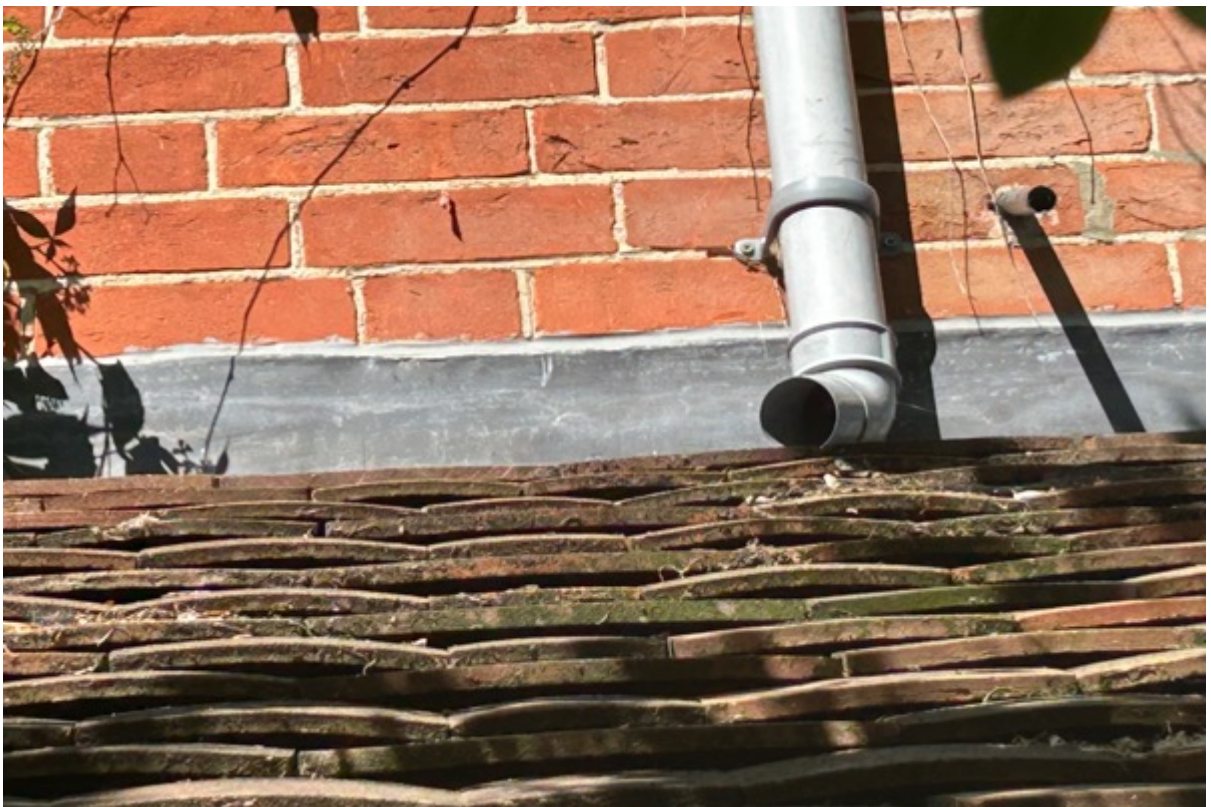
Flashing to the same subsidiary roof in satisfactory condition.
