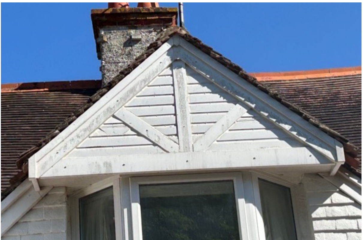
Front gable covered with PVC boarding in satisfactory condition.
