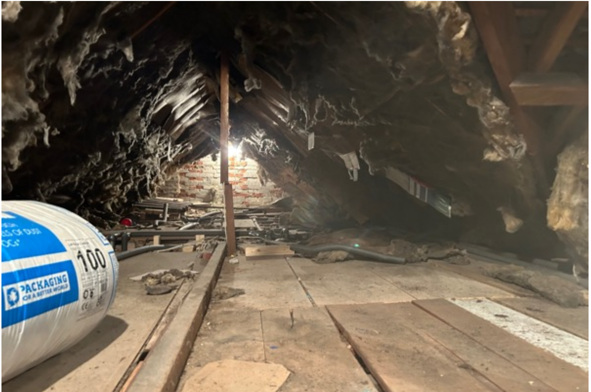
General view of the front-to-rear section of the roof space.
