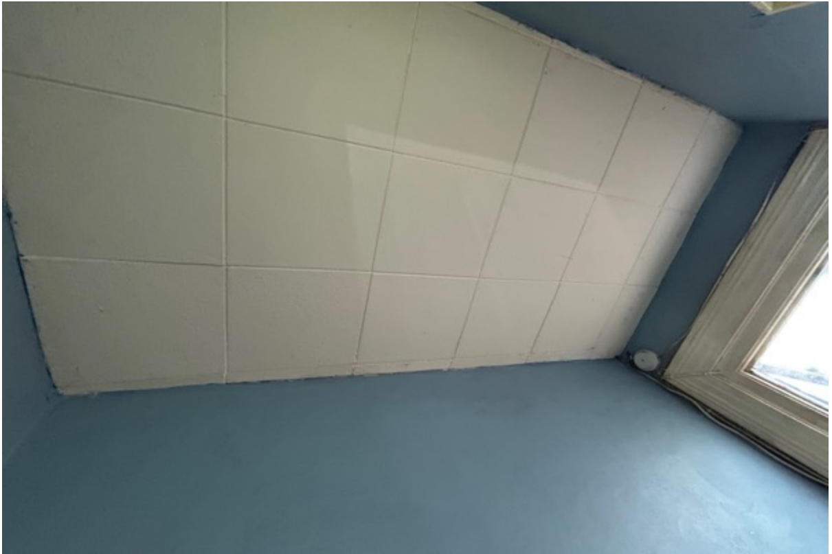
Polystyrene ceiling tiles to the rear lobby ceiling.
