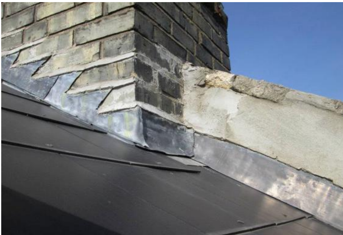
Correct flashing detail between slates and stack/parapet wall to right side of main roof.
