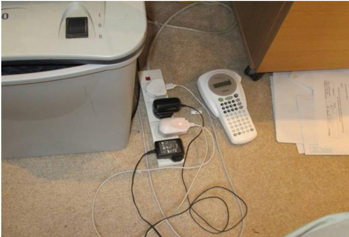
Extension cords to first floor centre bedroom suggesting inadequate power supply.
