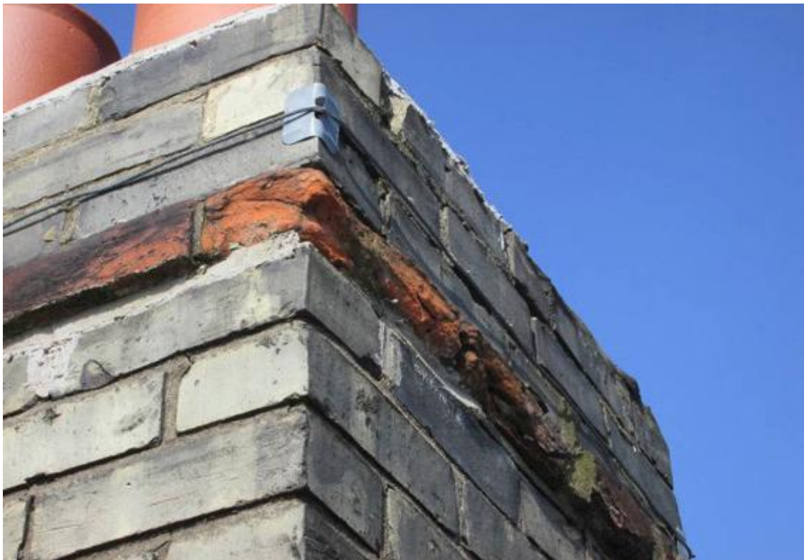
Chimney stack to main roof with bricks to ornamental red band starting to spall (2).
