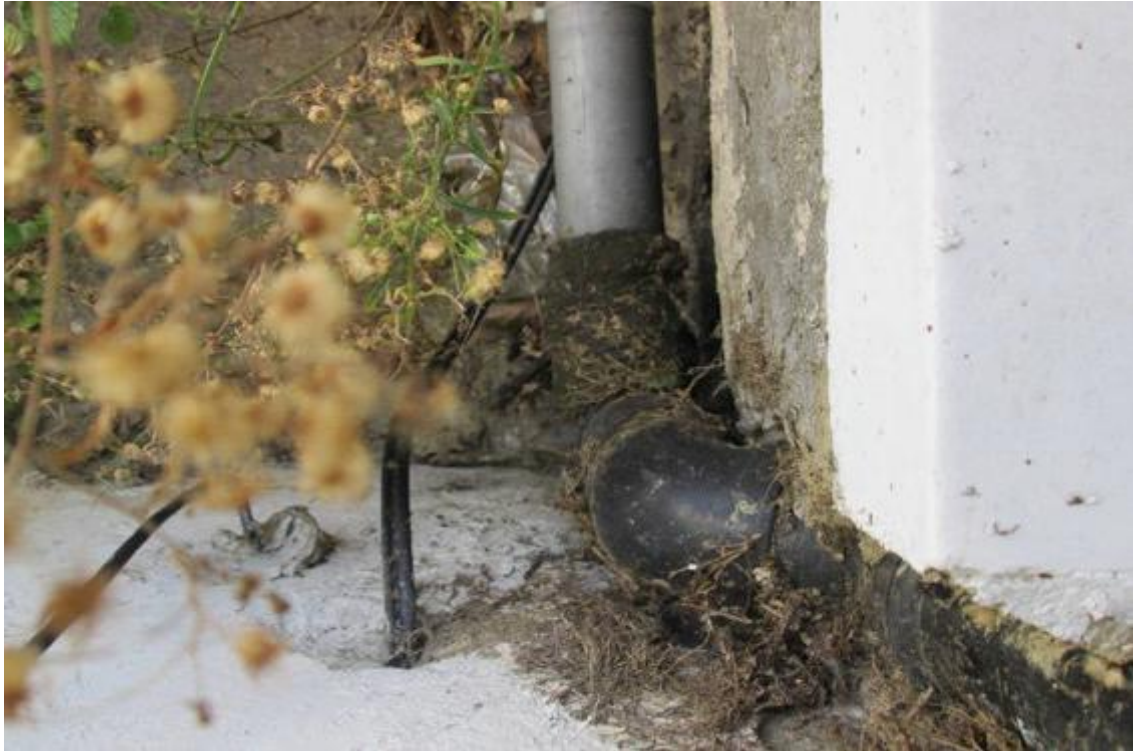
Bandaged joint at low level to downpipe to right side of front elevation.
