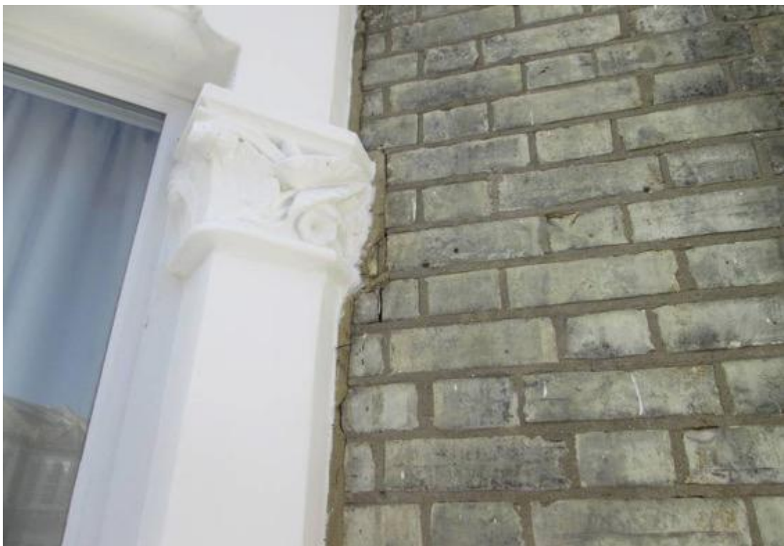
No separation between bay and front elevation.
