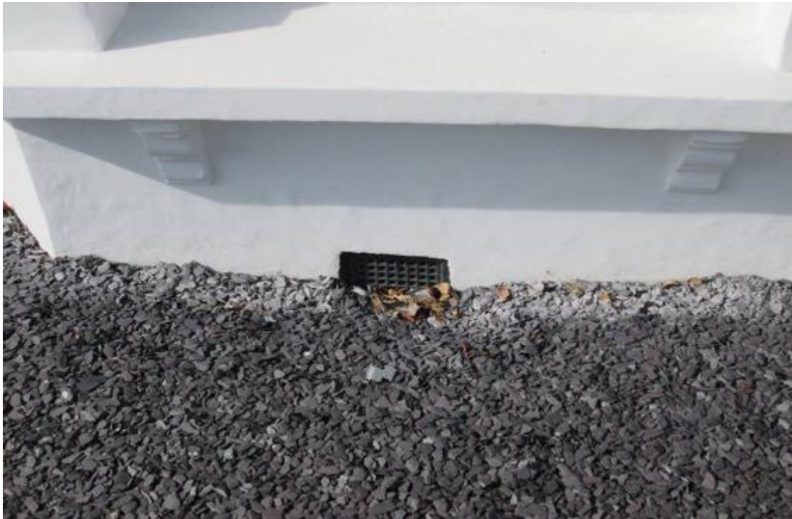
Vent at low level to front elevation.
