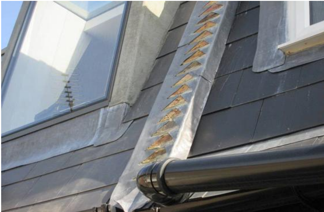
Parapet wall to rear left corner of main roof with good lead flashing protection.
