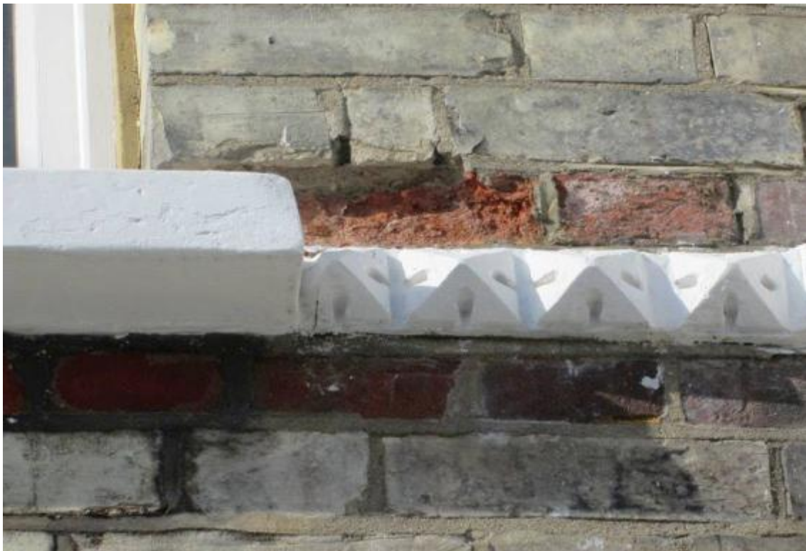
Single spalled brick at first floor level to front elevation.
