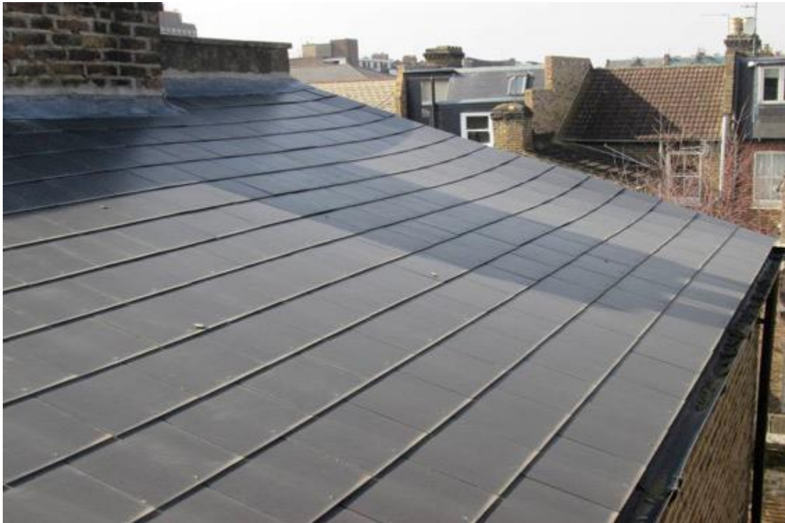
Uneven profile to slating to upper back addition roof.
