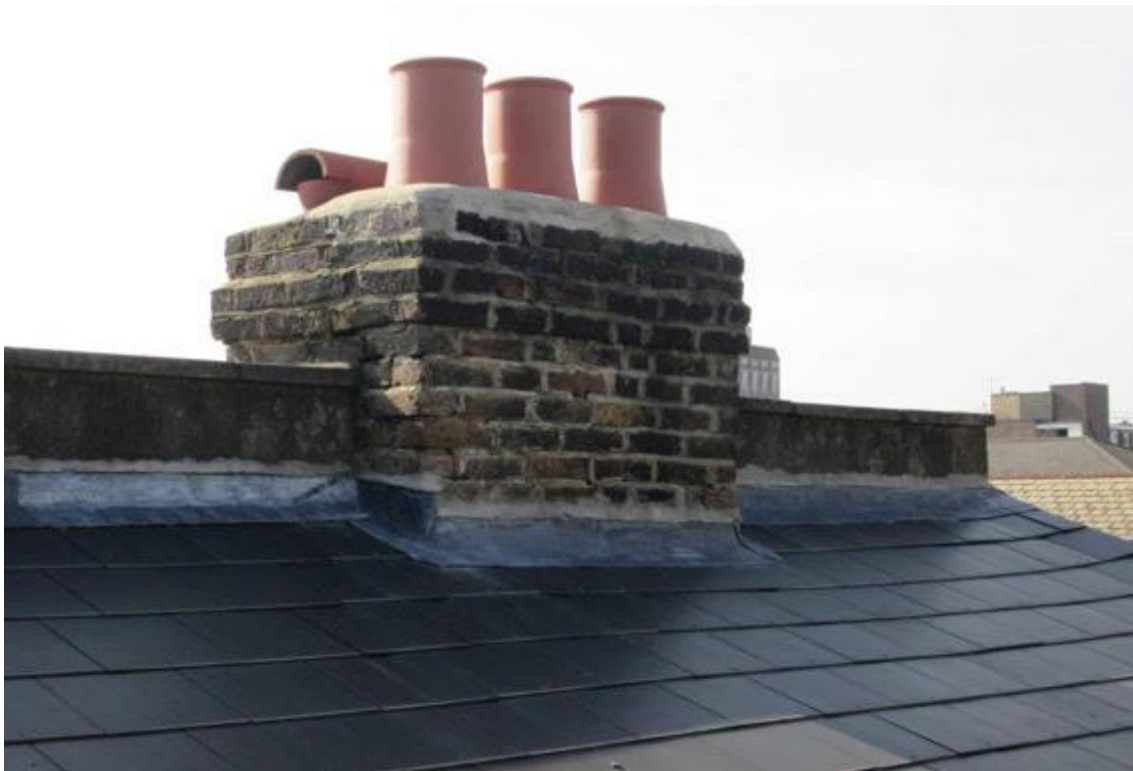
Untidy brickwork to chimney stack to left side of upper back addition roof.
