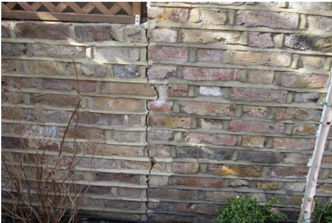
Crack to rear boundary wall.
