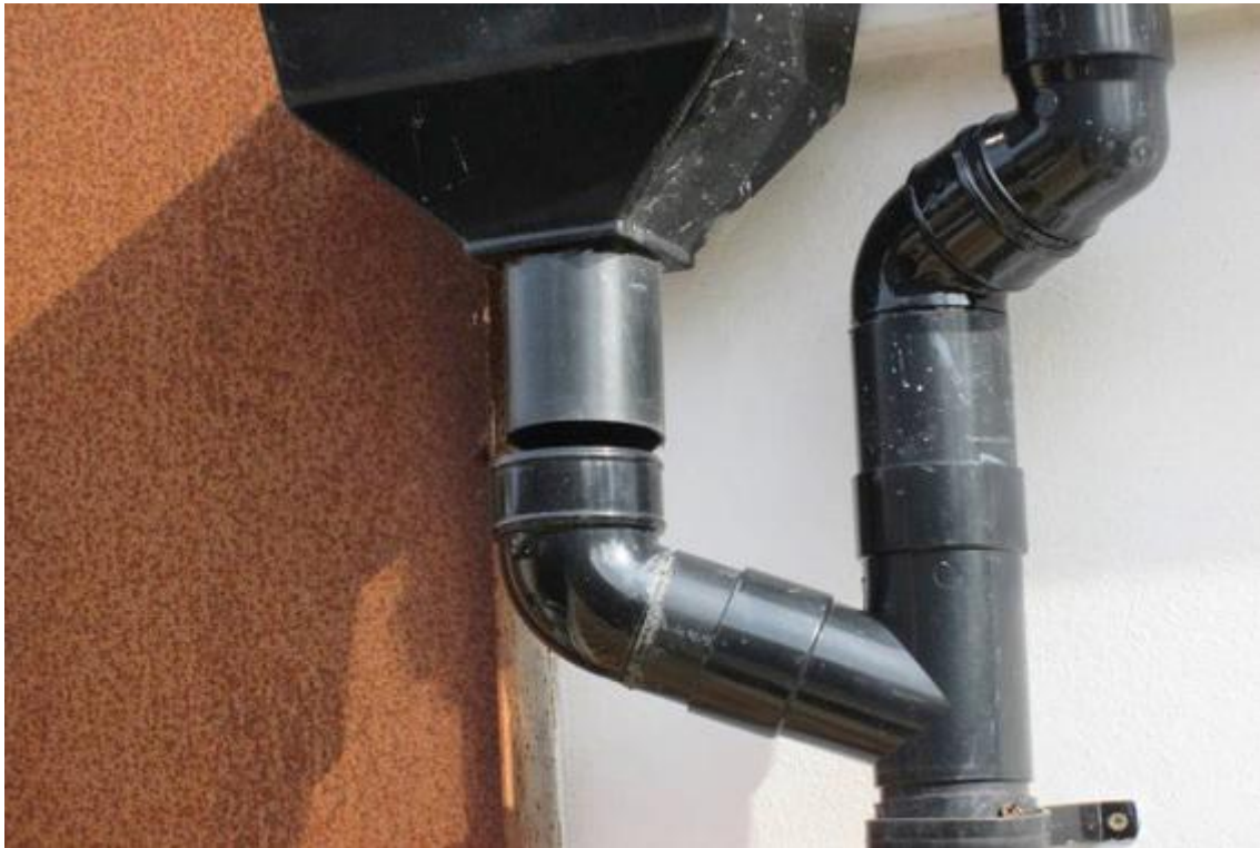
Separated joint between rear hopper and downpipe beneath.
