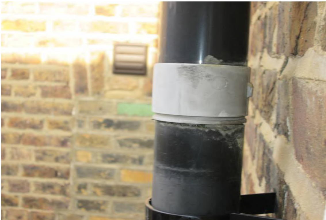
Weeping rear downpipe joint.
