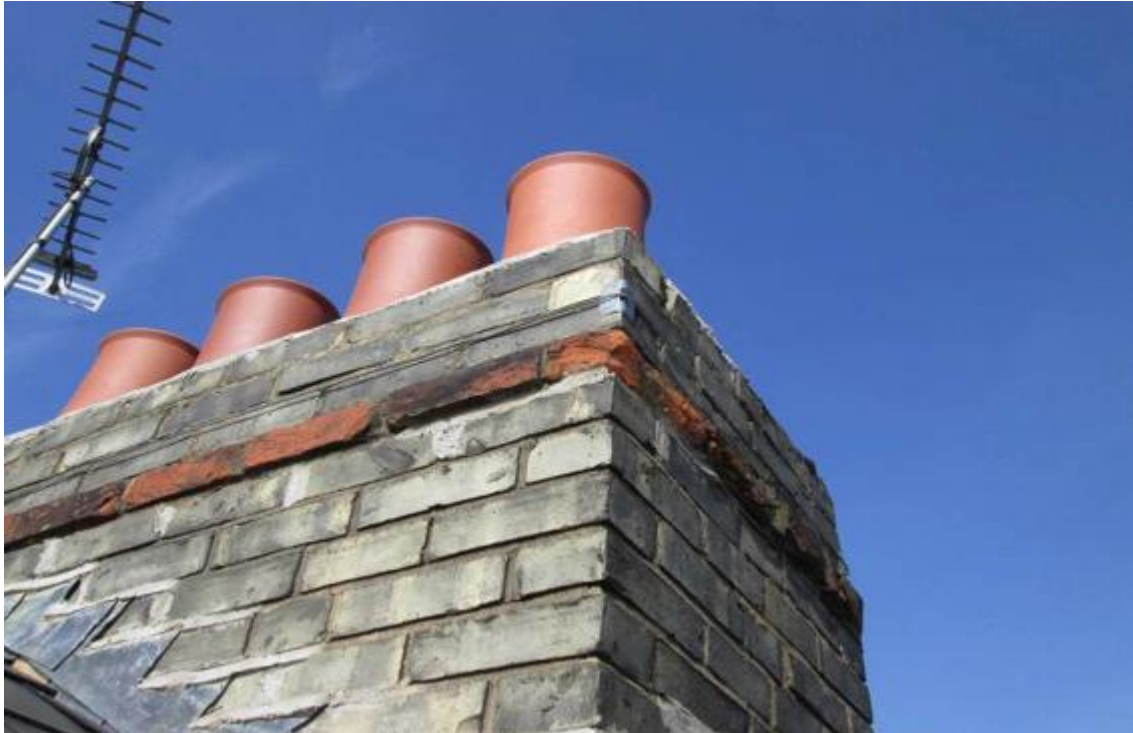
Chimney stack to main roof with bricks to ornamental red band starting to spall (1).
