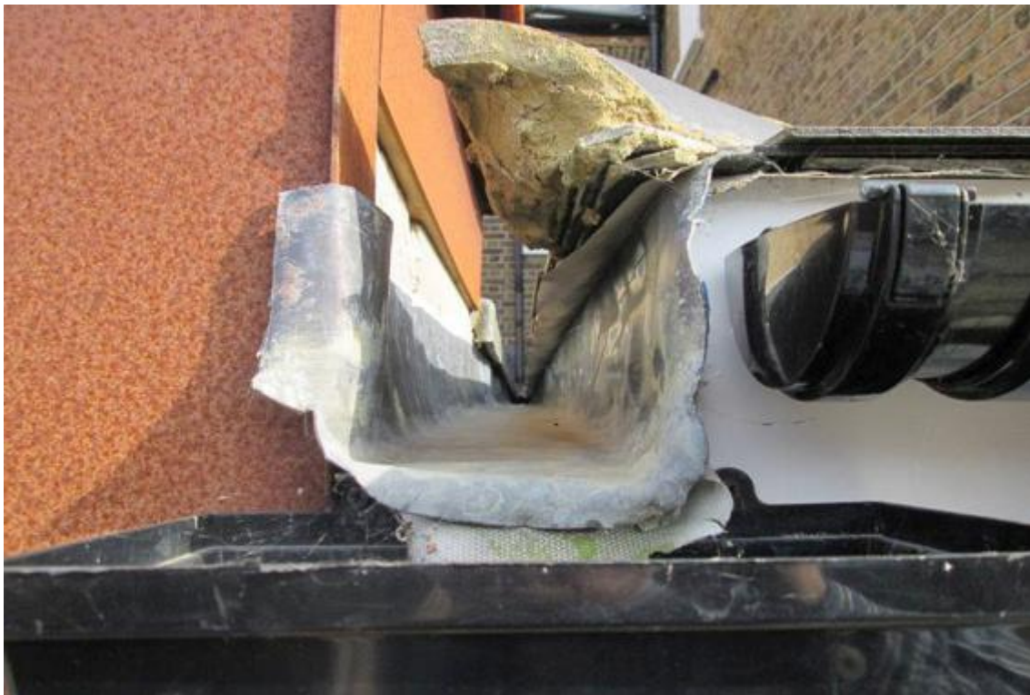
Rear end of box gutter draining lower rear subsidiary roof.
