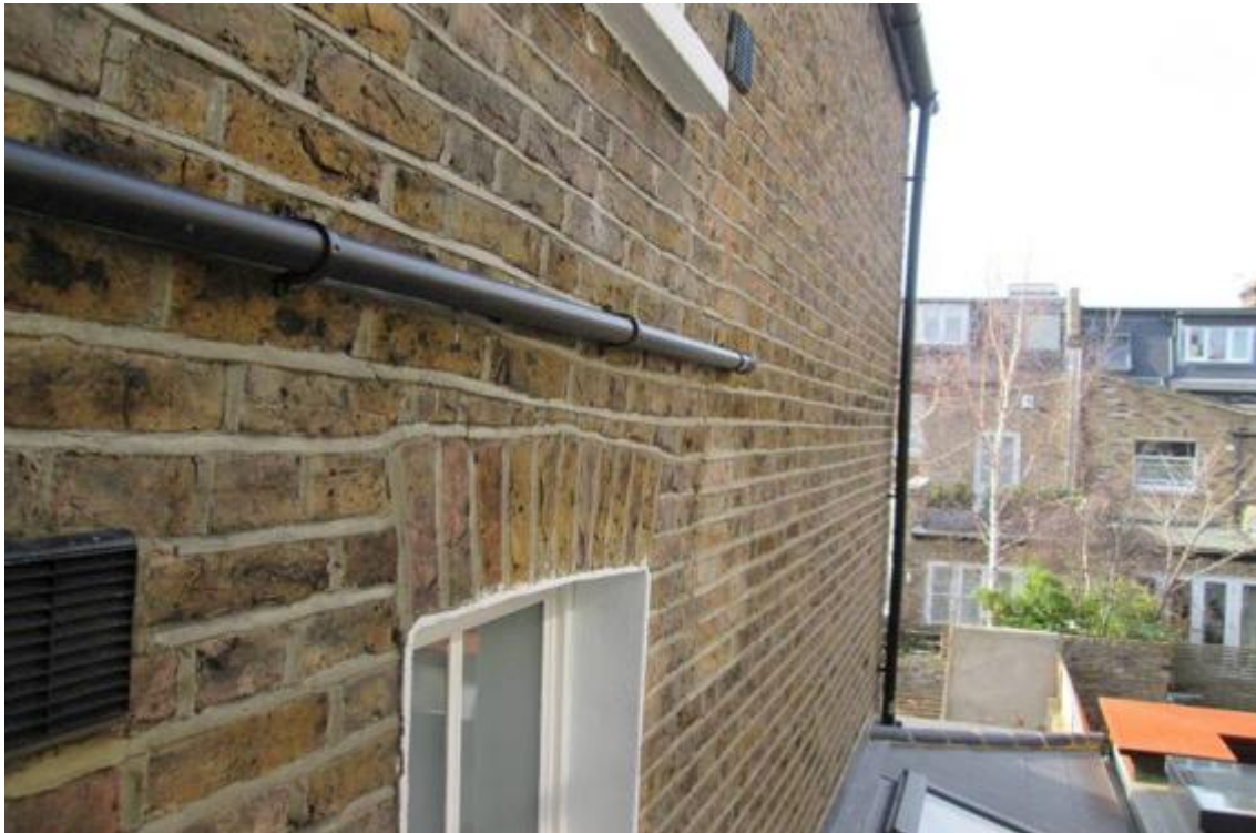
Brickwork slightly twisted over first floor bathroom window.
