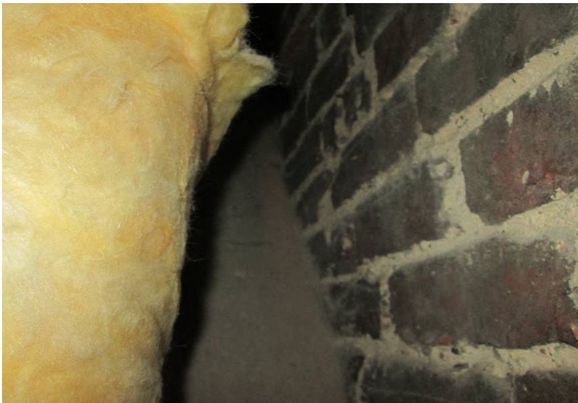
Open gap to right side of second floor bedroom.
