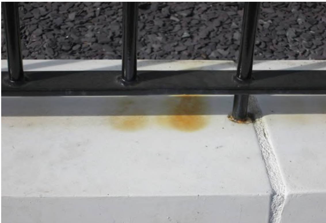
Rust staining to front boundary wall, due to bottom rail to front railings being unpainted.
