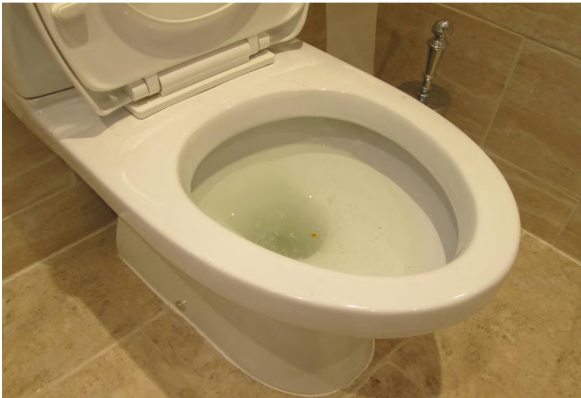
Water at top of bowl to first floor WC pan.
