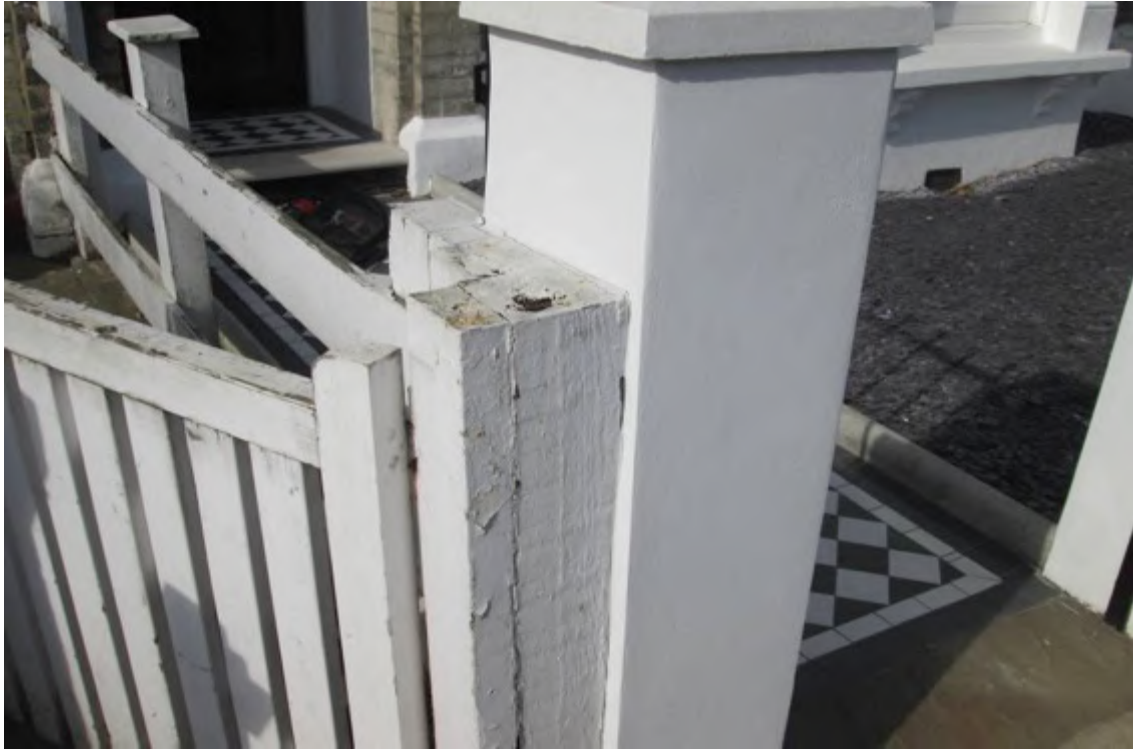
Render to garden gate pier will be unfinished behind timber post.
