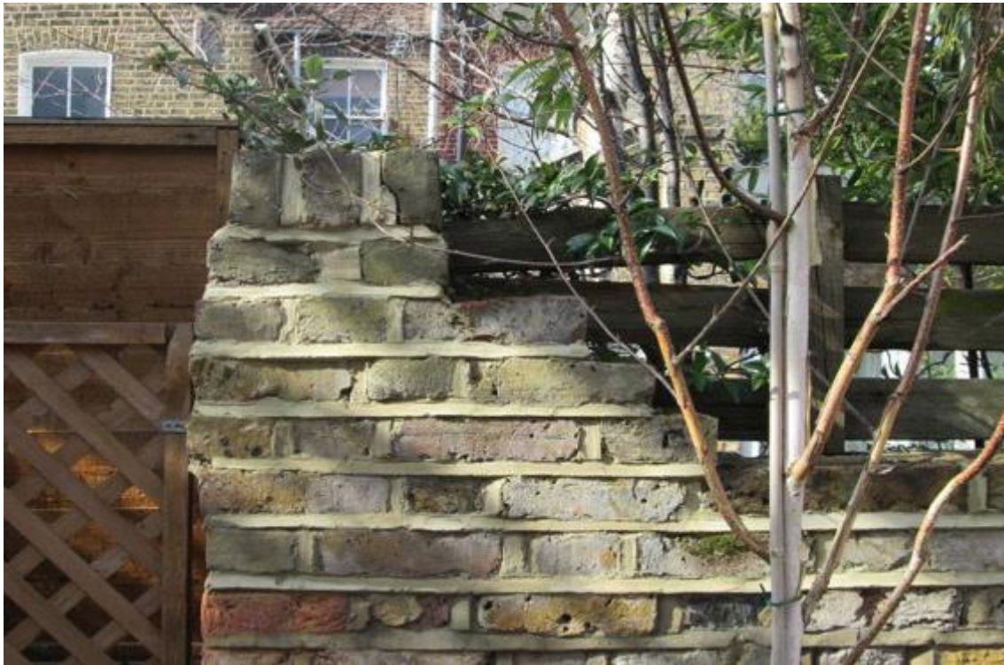
Incomplete high-level brickwork to rear boundary wall.
