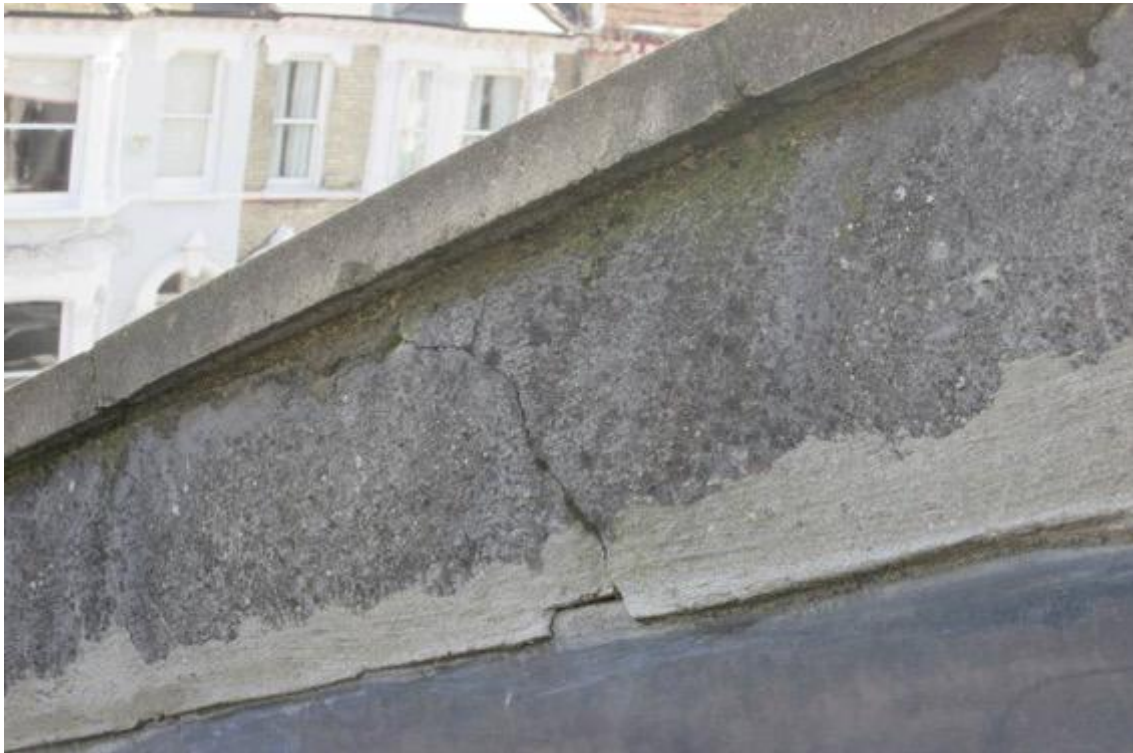
Crack through render to parapet wall to left side of main roof.
