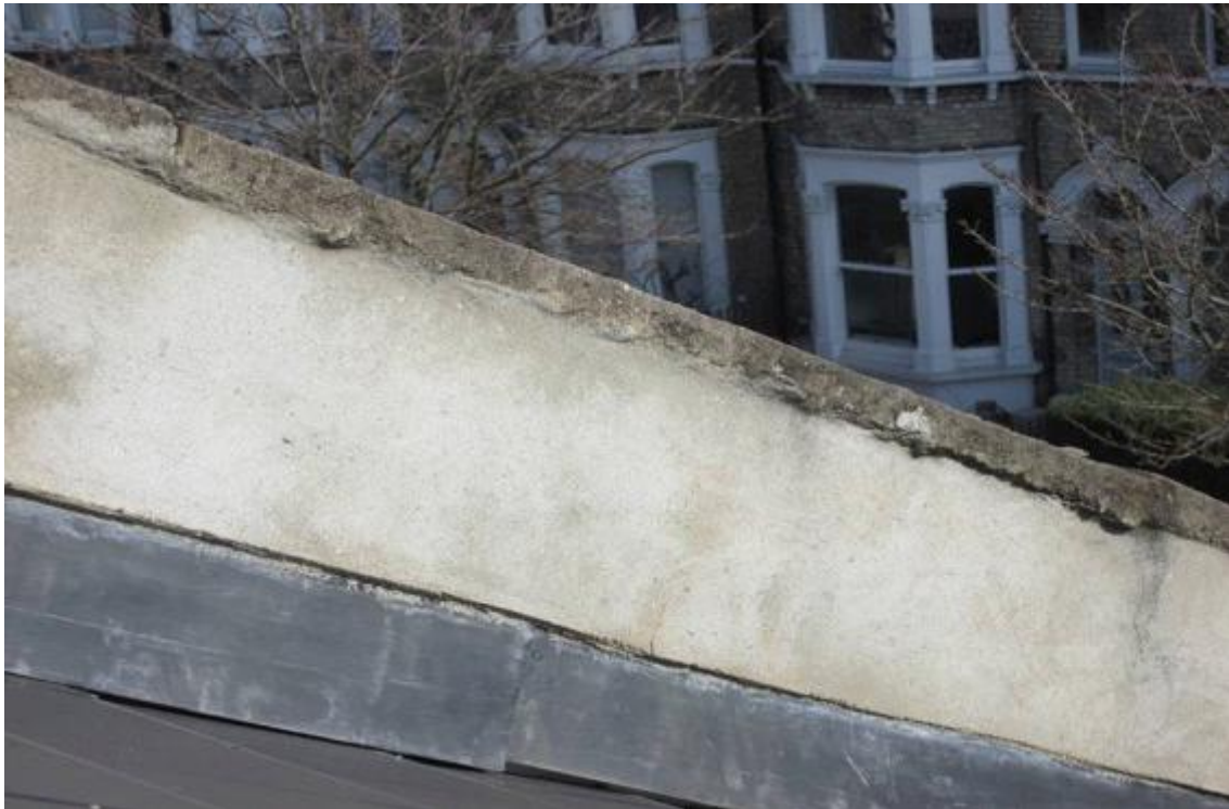
Parapet wall to right side of main roof with no oversailing capping detail.
