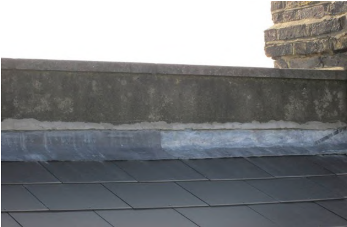
Parapet wall to upper back addition roof with poor capping detail but correct flashing detail.
