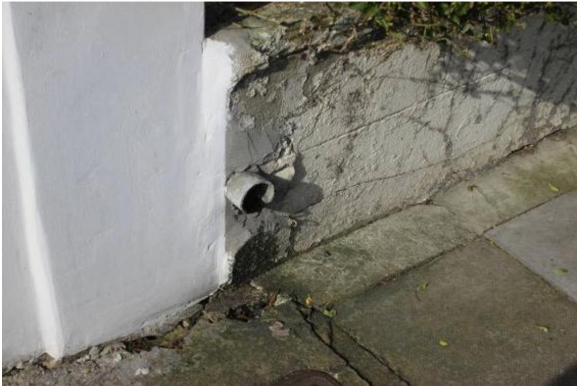
Rainwater downpipe discharging onto pavement.
