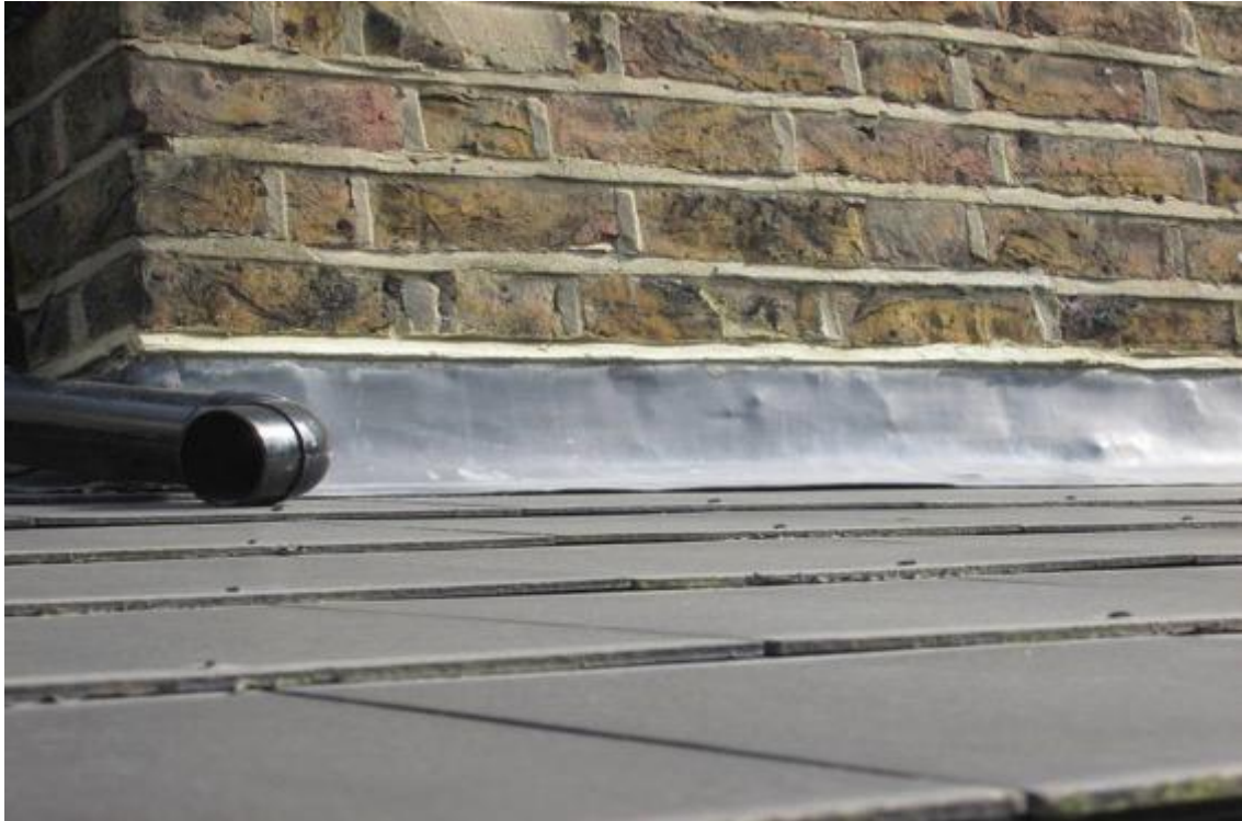
Correct flashing detail to lower rear subsidiary roof.
