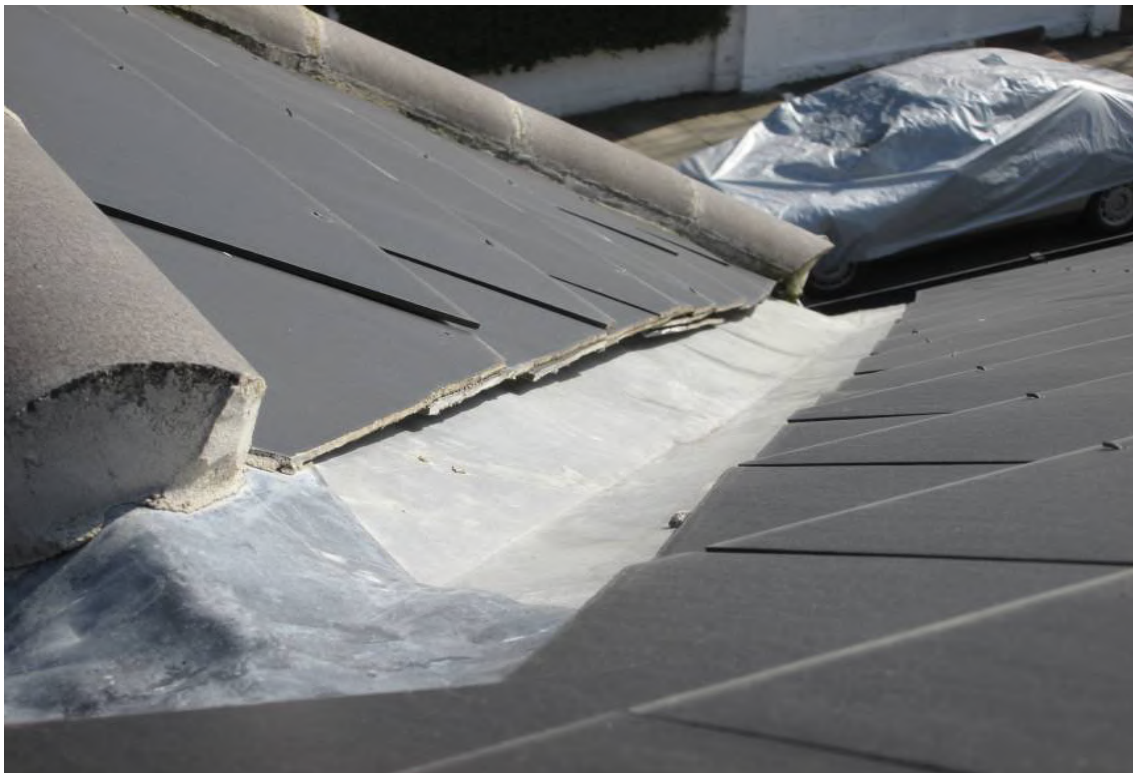
Valley gutter to front of main roof covered with leadwork.
